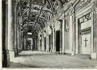
INTERIOR OF THE PORTICO, ENTRANCE TO ST. PETER'S
