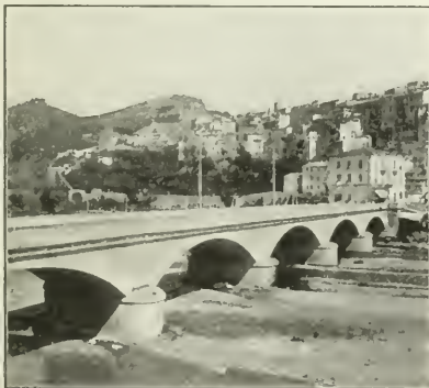
BRIDGE AND PORTION OF THE OLD CITY, VENTIMIGLIA
